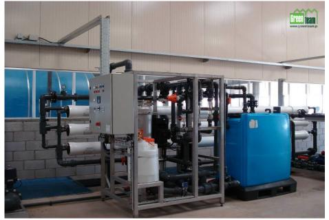
Reverse osmosis installation with a capacity of 360 m³/day. Desalination of min. 98% of well or mains water. Complete with a.o. conductivity meter (EC) and timer for automatic production of water at off peak hours.
